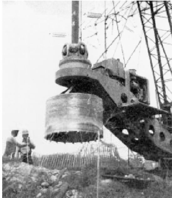
Figure 4-3 — Core Barrel for Rock Drilling
